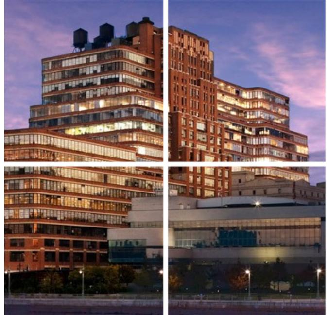
Starrett Lehigh is the eighth largest office building in NYC at over 2.3 million square feet. A pre-war building constructed in 1931, the building is heated by steam radiators fed by two-pipe steam distribution. Tenants provide their own water-cooled package units, connected to central plant cooling towers. In 2012, the base building controls were unfortunately destroyed by Hurricane Sandy, but it created the opportunity for new solutions.
